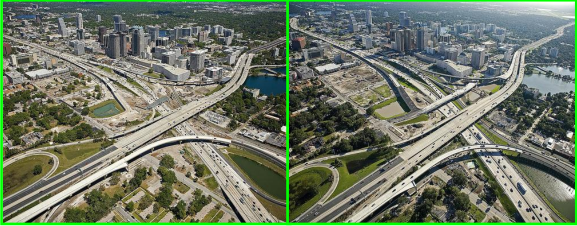
Figure 27: Downtown Construction - February (left) and August (right) (trans4mation.org)
